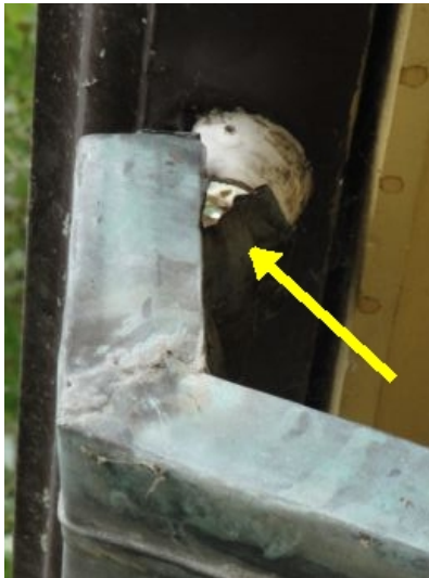
Disconnected downspout
