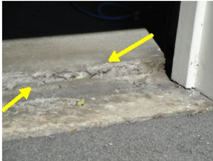
Settlement crack
